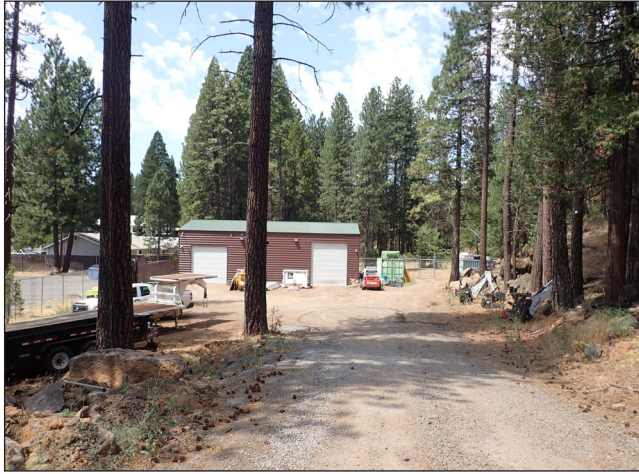
PHOTO 1: APN 028-170-015-000 Maintenance Building with Equipment
