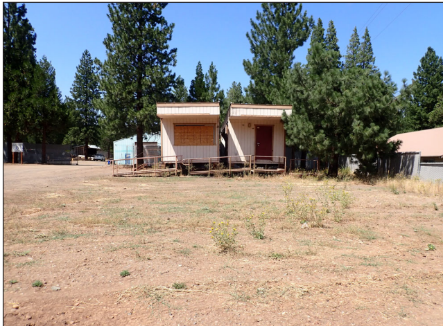
PHOTO 5: APN 028-410-018-000 Temporary Buildings
